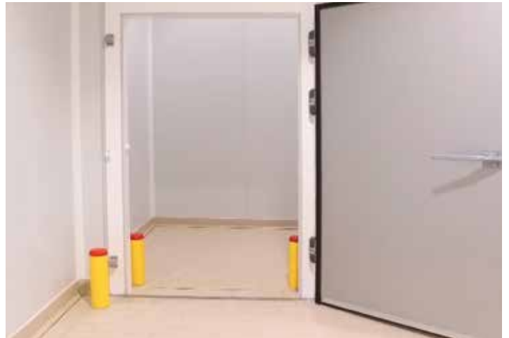
Bollards for protection of shelves and doors
